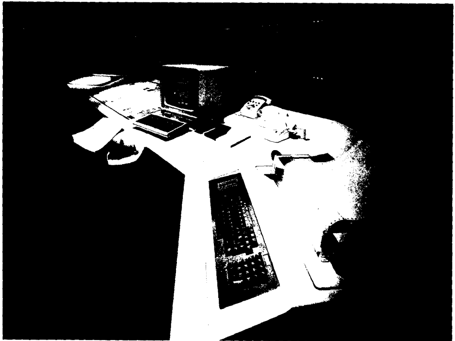
Electric installation, control and transformation centre of the Banco Hispano Americano building, Las Rozas, Madrid.
