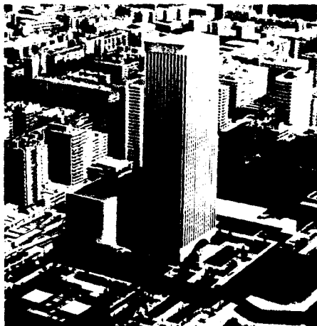
Security and control installation in the Torre Picasso building, Madrid
